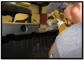
58. Once you have made sure the plate fits correctly with the snorkels, go ahead and attach the plate with three **T141** screws.
