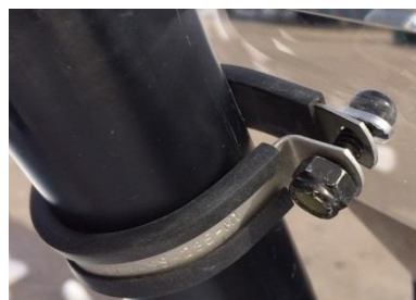
Clamp installation detail
