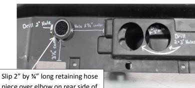
piece over elbow on rear side of panel. Install hose clamp and tighten.
