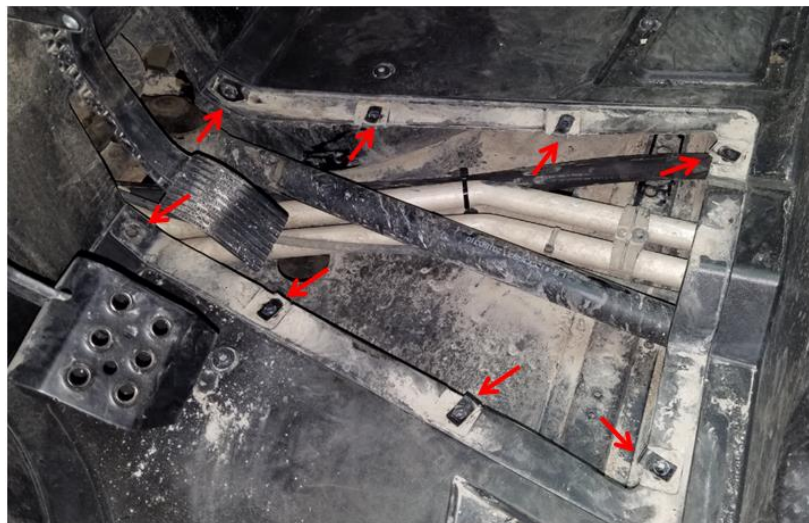
Figure 1 – Front Tunnel Cover Removed
